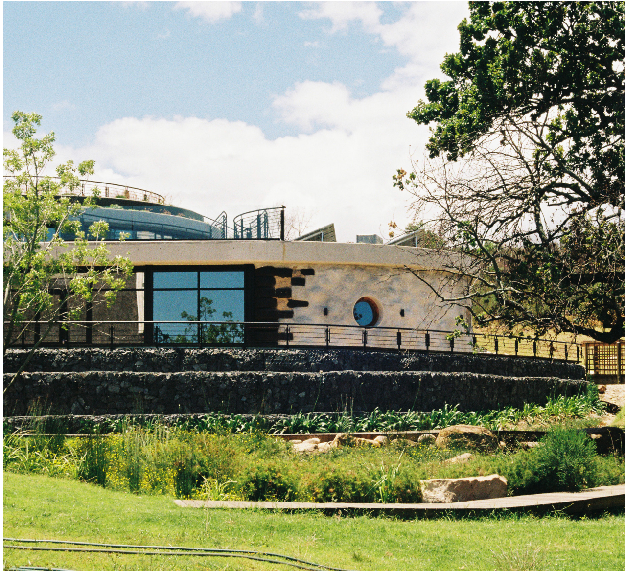
A NEW POND - excess water from the black water treatment system & rainwater harvesting allowed the team to create a wetland pond next to the facility. This allows for more accessible of environmental education about those biomes
